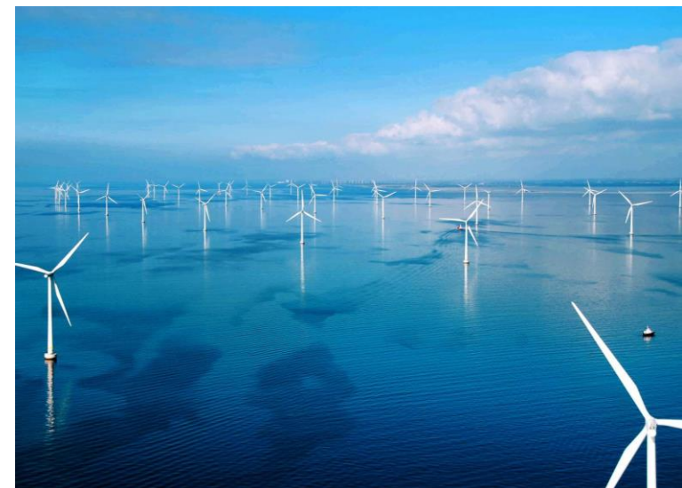
Rødsand 2 Offshore Wind Farm, Denmark
